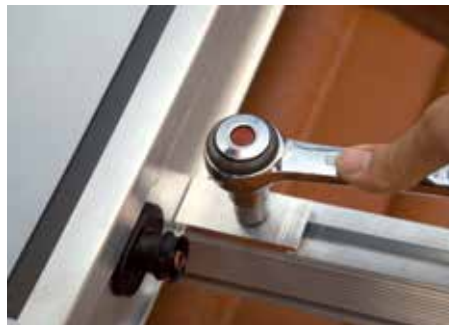
Fixing of collector to rail
