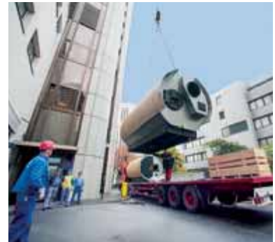
Delivery of a Vitomax boiler to site
