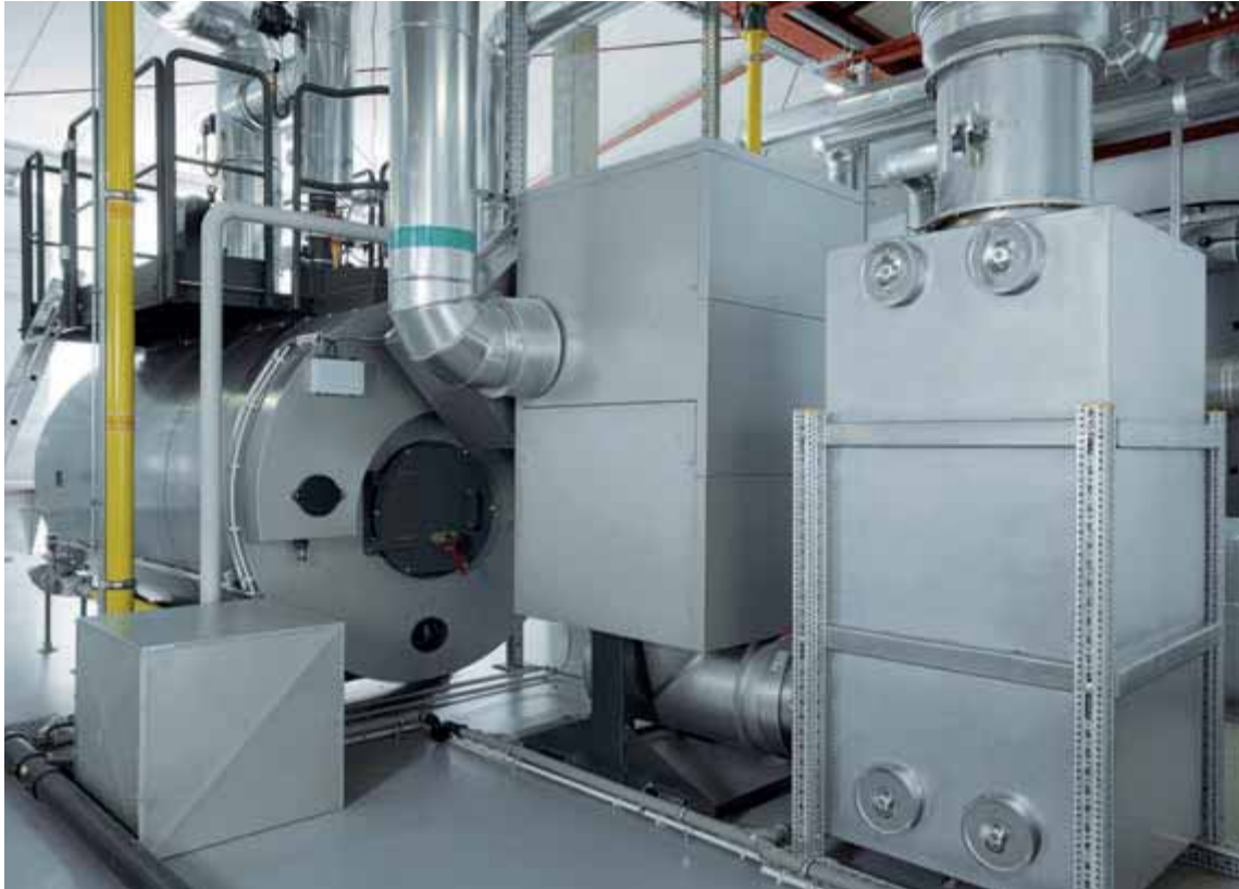
The Vitotrans 300 flue gas/water heat exchanger draws heat from the Vitomax boiler's hot flue gases and so improves efficiency.
