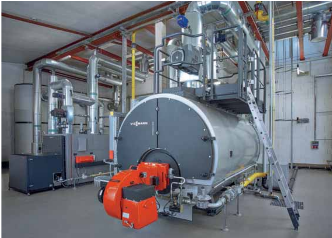
Vitomax LW hot water boiler (2300 kW) and Vitoplex 200 low temperature boiler (700 kW)
